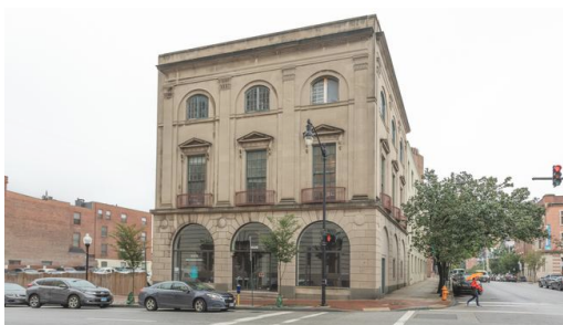
Agora Cos., a Baltimore-based international publishing company, just settled on this three-story historic building in Mount Vernon for $5.75 million.
